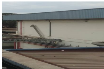
Godown 7 & 8 - Metal Cradling & Roof Capping Damaged
