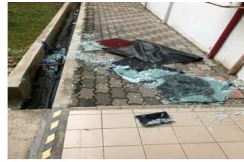
Side Entrance to B Block - Broken Glass Door
