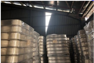
Godown 7 & 8 - Metal Cradling & Roof Capping Damaged
