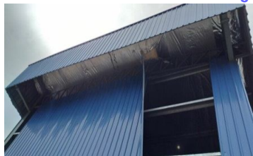
Phase 2 Beam Stocker Building - Metal Tilt Cradling Flied Off
