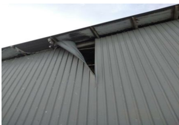
Godown 7 & 8 - Metal Cradling & Roof Capping Damaged
