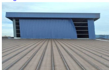
Phase 2 Beam Stocker Building - Metal Tilt Cradling Flied Off
