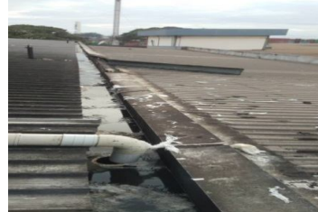
Phase 1 & 2 Building - Joint Metal Capping Between Buildings Flied Off
