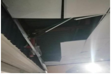
In Front of Guard House - Ceiling Board Broken and Flied Off
