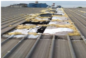
Phase 2 Beam Stocker Building - Metal Tilt Cradling Flied Off
